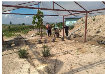
Construct Storehouse for seedling at LKK
